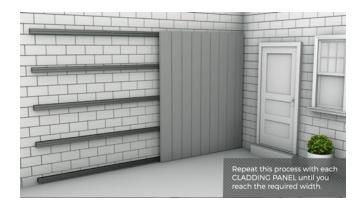
It is possible to fit your Boards side by side by simply butting the two ends up together. You may need to install more Battens if you wish to do this, as each Board will need to be supported on a Batten where it meets the next Board. Continue to fit the Cladding Boards in this manner until you have completely covered the area you want.
